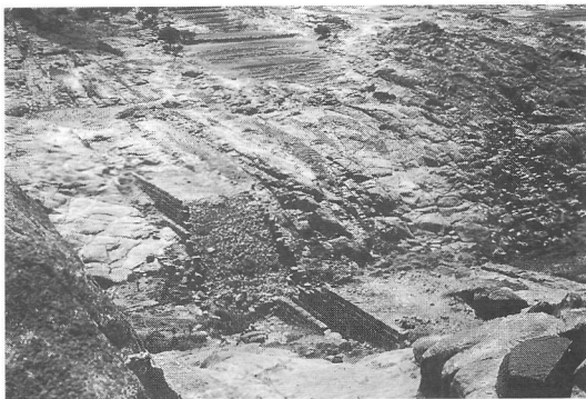
Figure 4. Major Himyarite dam of Sedd al-Ajmar, near Khirbet Maryah
